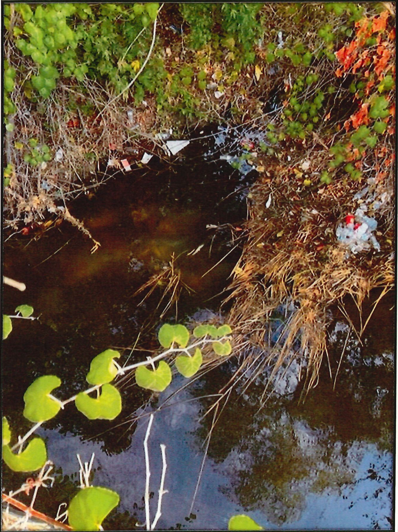
Stormwater Inspection of Outfall MC_005 on the far west side of campus on 09.19.2023. Another view of debris in stream adjacent to the IM field where the trash bins are overflowing.
