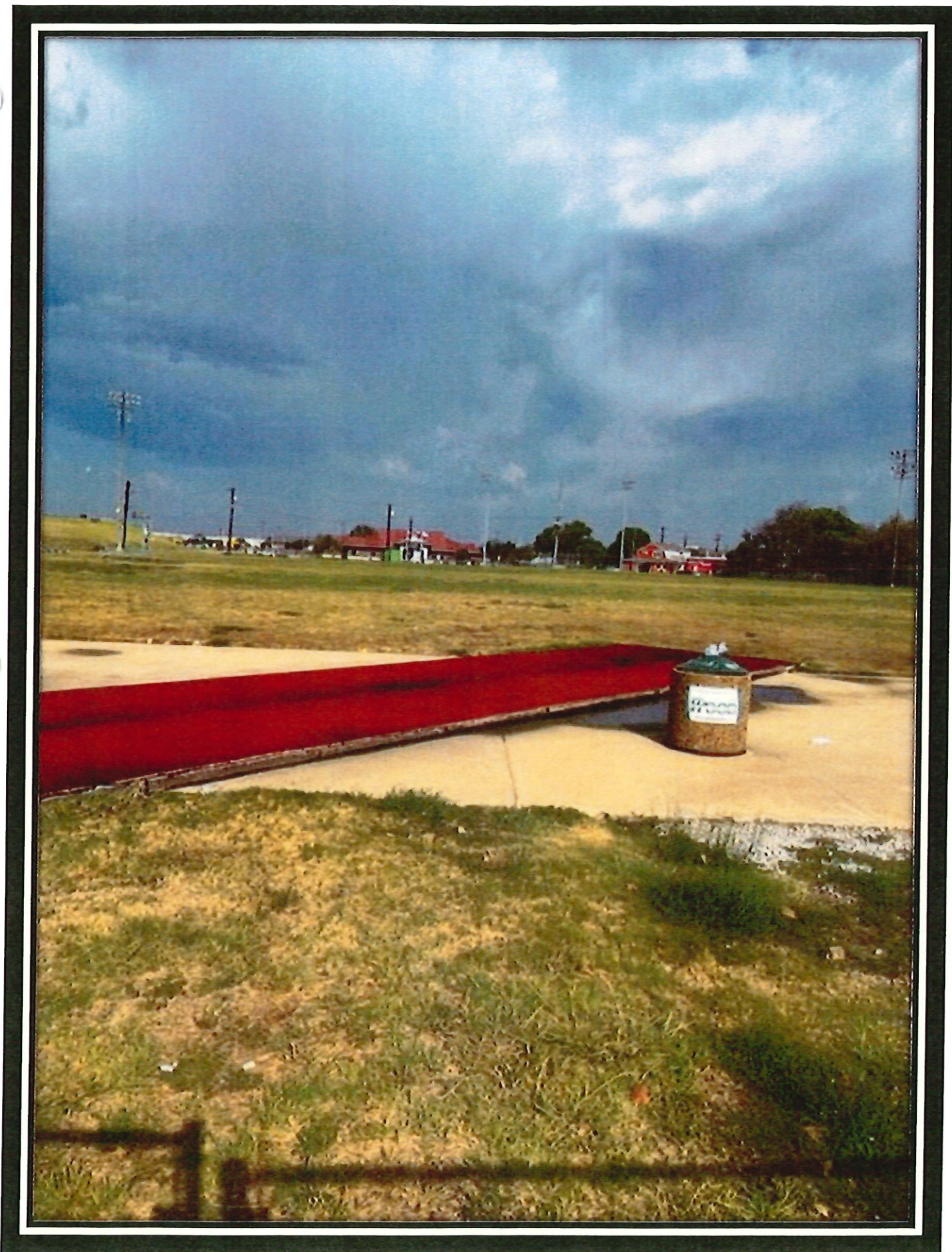
Stormwater Inspection of Intramural Field adjacent to MC_005 outfall on 09.19.2023 20 158 showing plastic bottles overflowing the trash bin. Plastic bottles are impacting the stream at MC_005.
