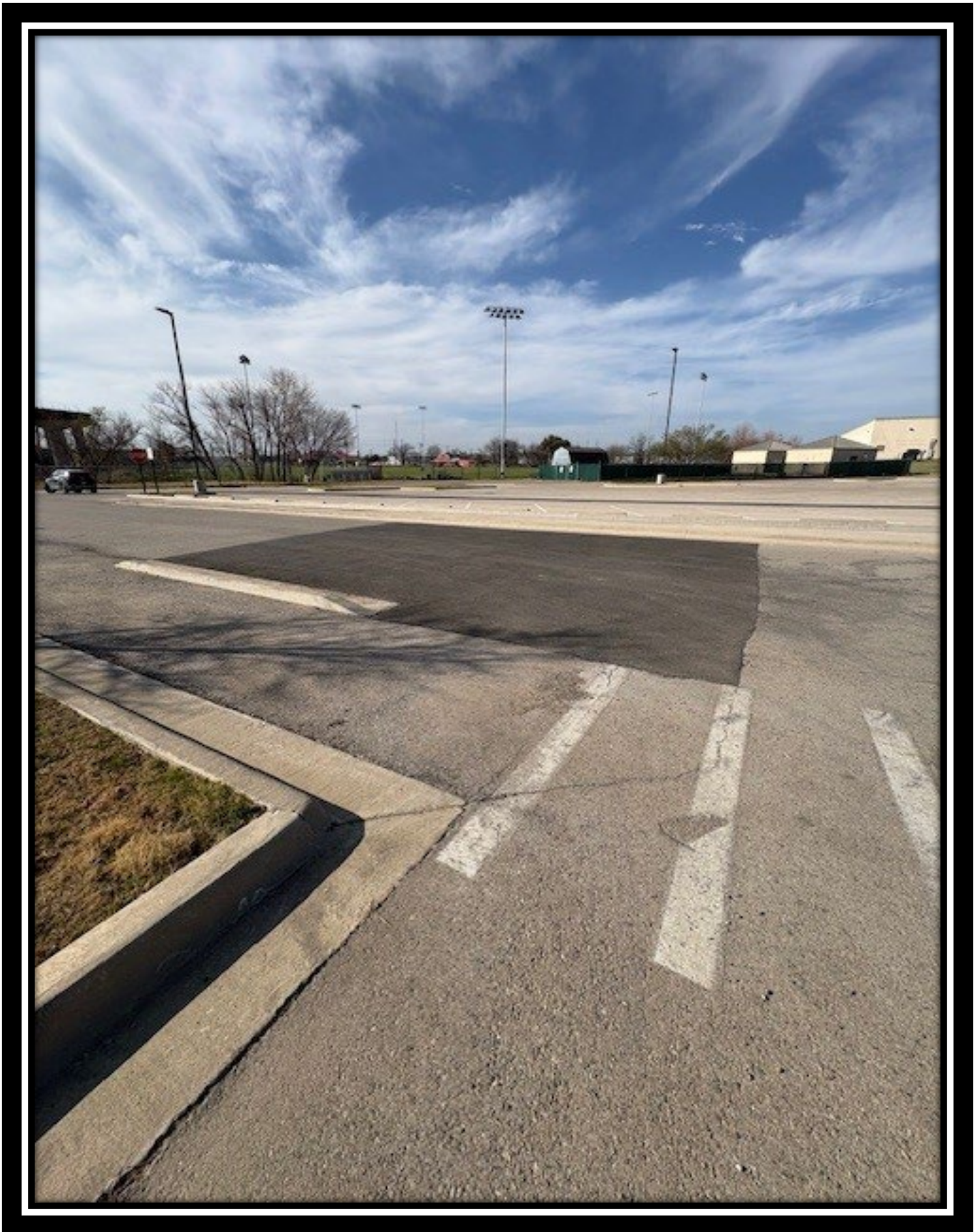
Sanitary sewer line repair completed in summer 2025 in Parking Lot 20.
