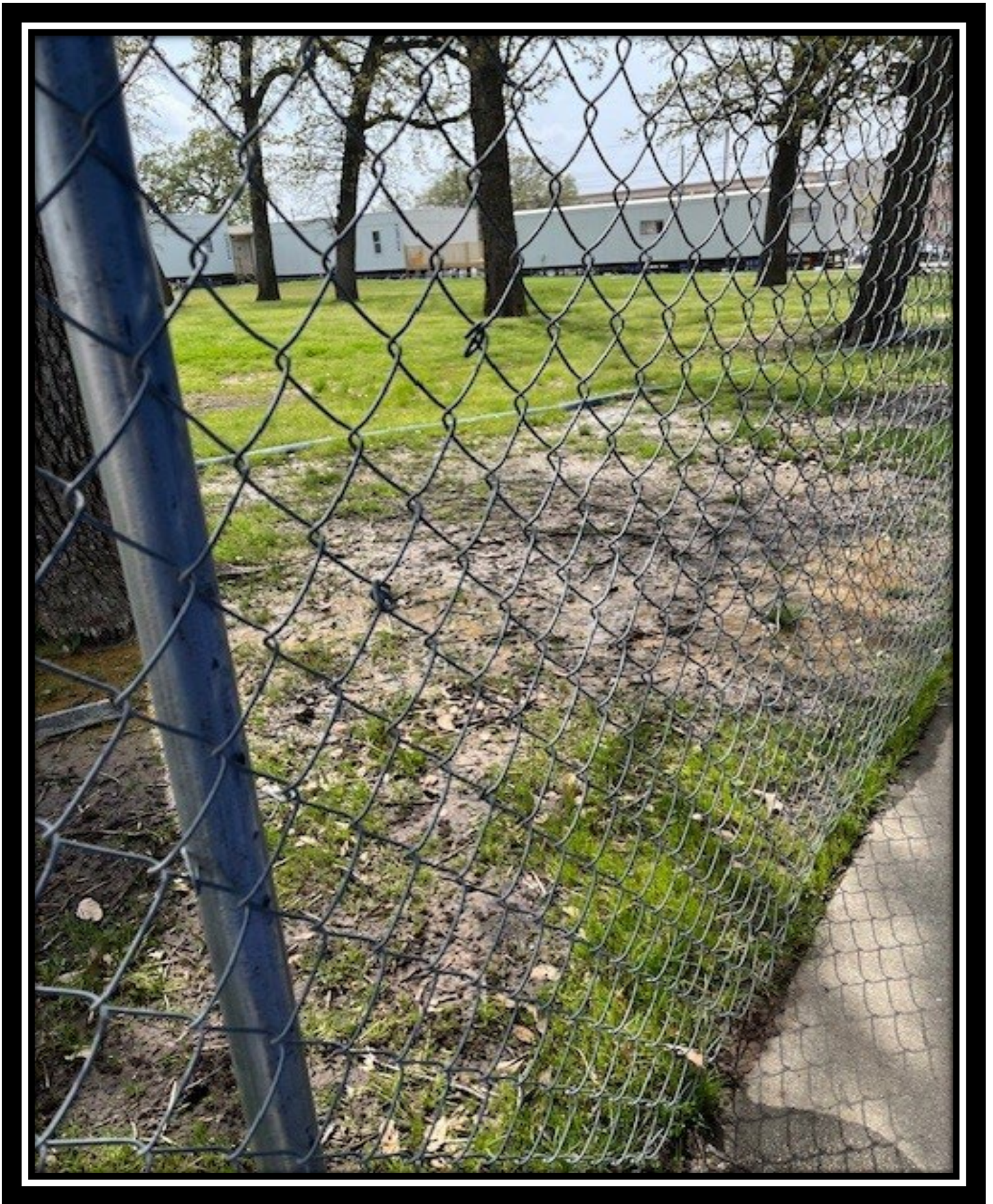
3-inch diameter blue hose dewatering construction pit for new Science and Technology building construction site. EHS asked the construction project manager to allow the pit water to infiltrate onto the ground surface rather than onto the sidewalk and Mulberry Avenue (April 2025).
