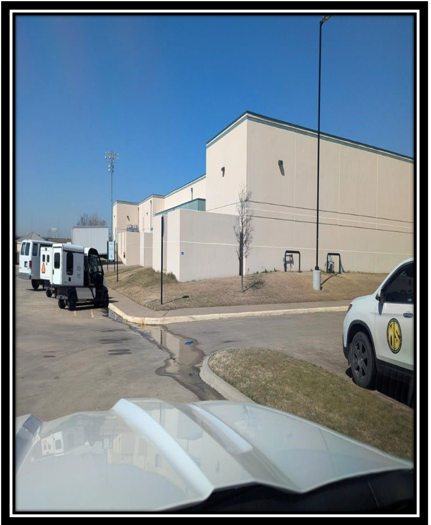
Broken water sprinkler runoff from Traditions Band Practice field (February 2025).
