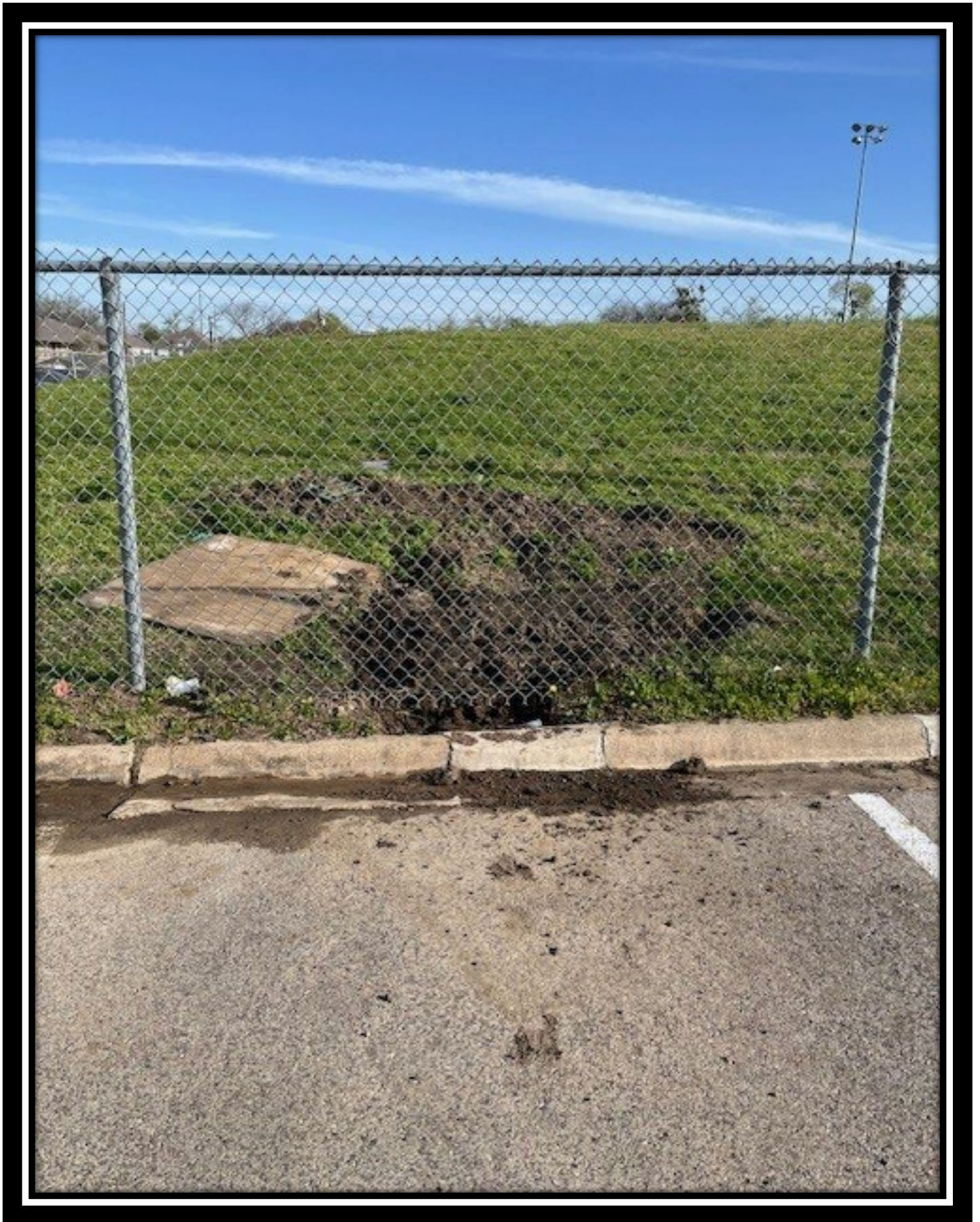
Repaired broken water sprinkler on Traditions band practice field. (March 2025)
