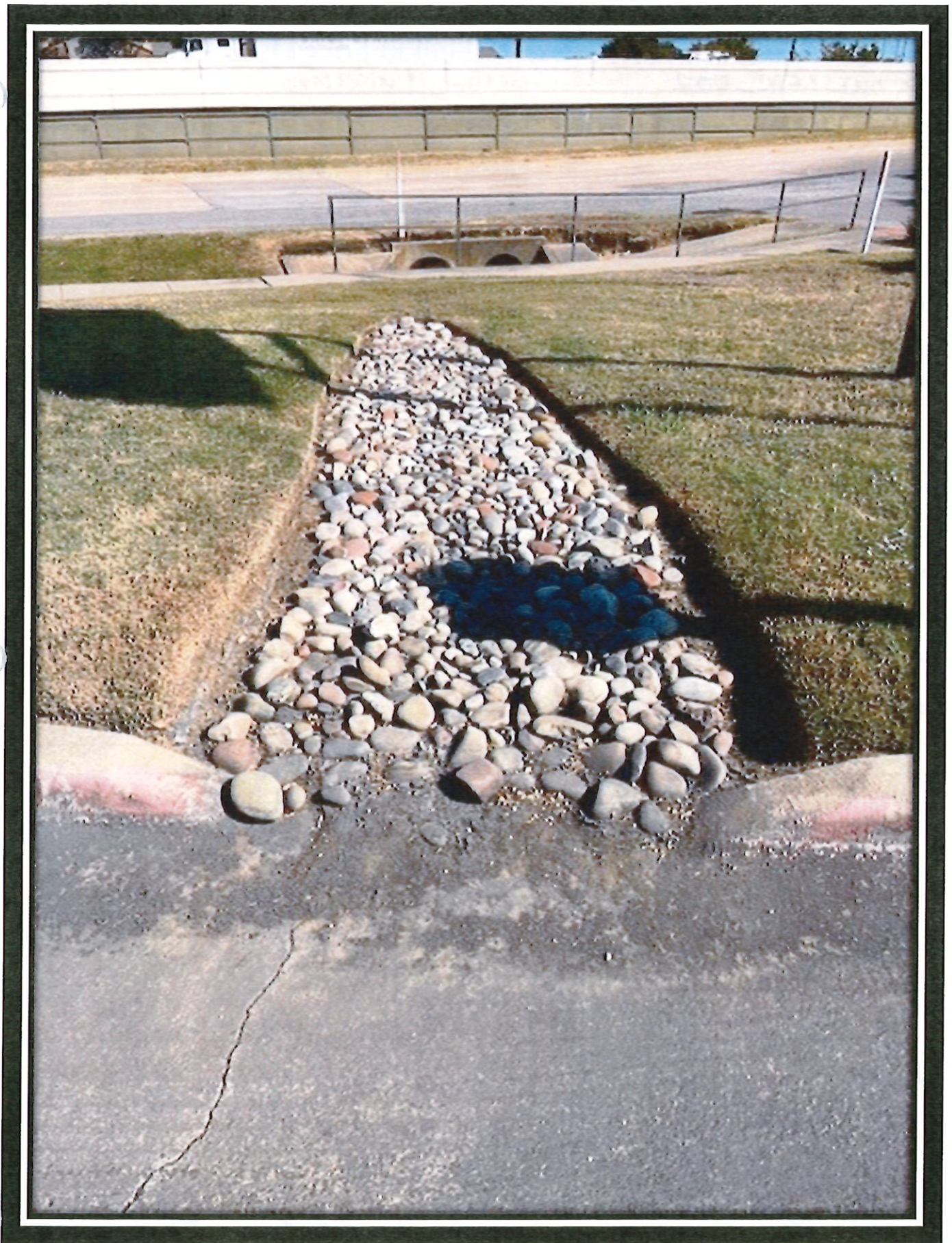
OUT_KFAC_001: Sloped outflow from the parking lot of Kristin Farmer Autism Center. Flow is toward the northeast and into the large culvert under the IH-35E frontage road shown in the background.
