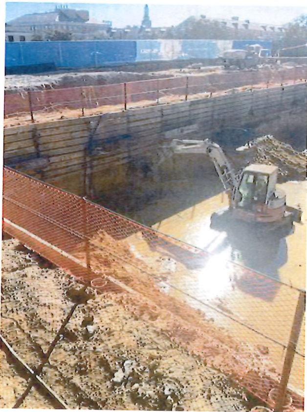
Berkel trimming soil to piling for lagging Ed Carrigan Nov 21, 2024 10:26 AM
