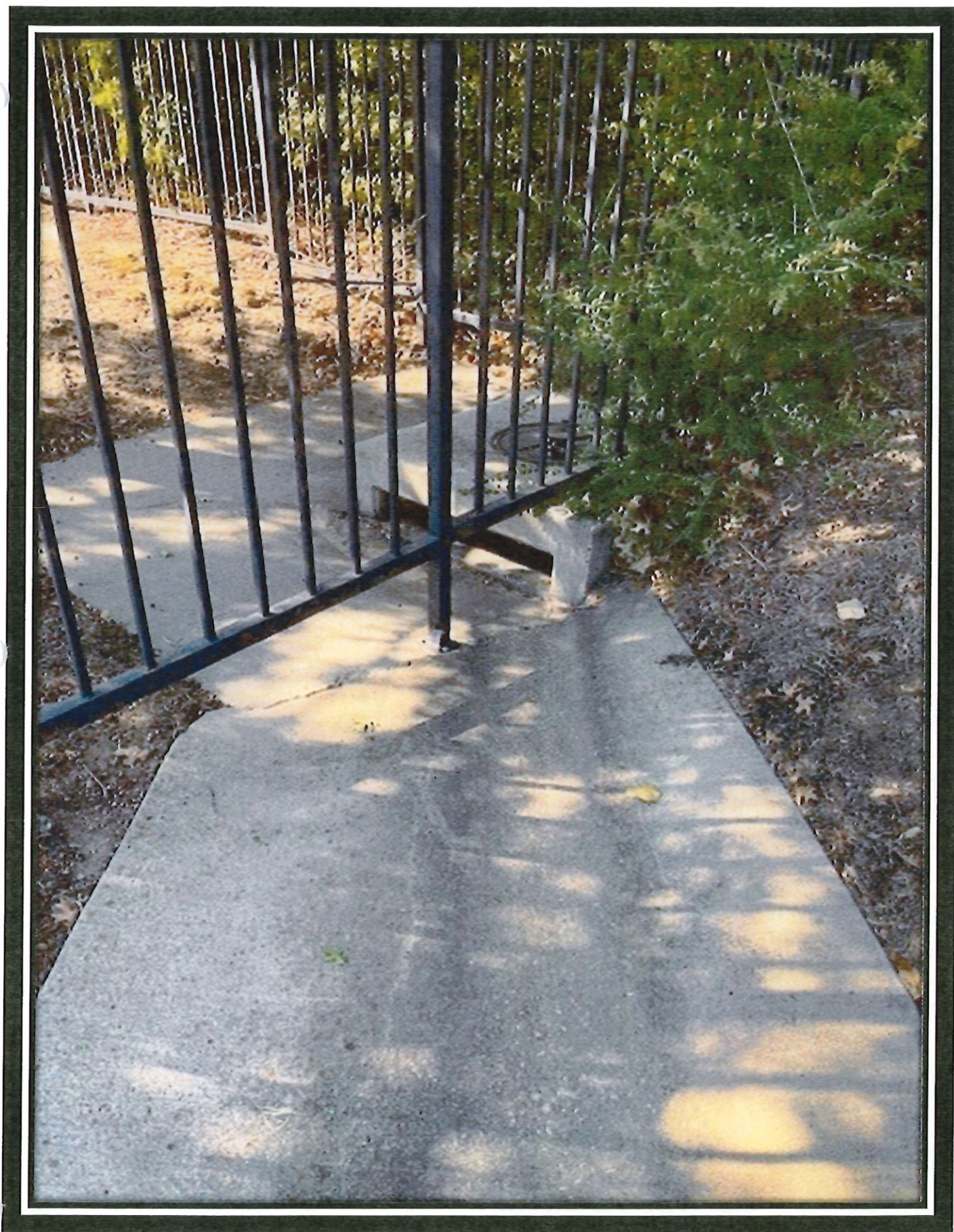
OUT_KFAC_002: Stormwater drainage under the fence at the northwest corner of the property and into the large box culvert.
