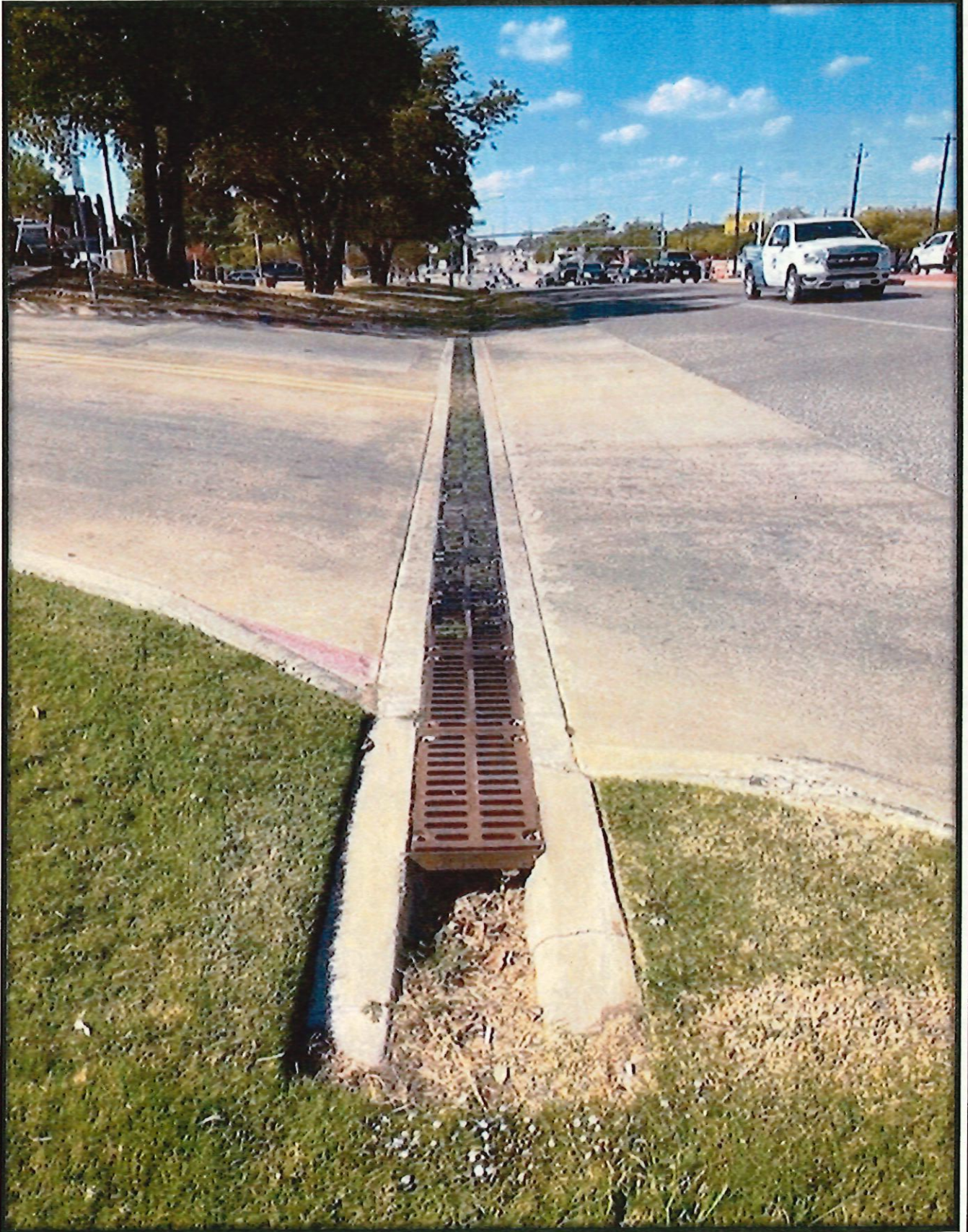
OUT_WHSQ_003: Stormwater drain on the north side of Woodhill Square where stormwater enters into the storm grate and travels parallel to Dallas Drive and into an unlined conveyance and into Fletcher Branch and then into Hickory Creek. View is to the west along Dallas Drive.
