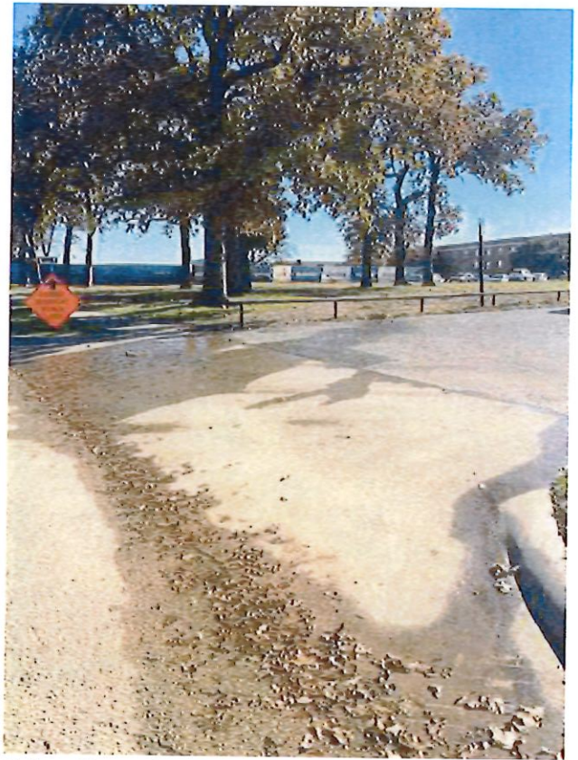
Outflow of Dewatering on NE Corner of Lot 7
