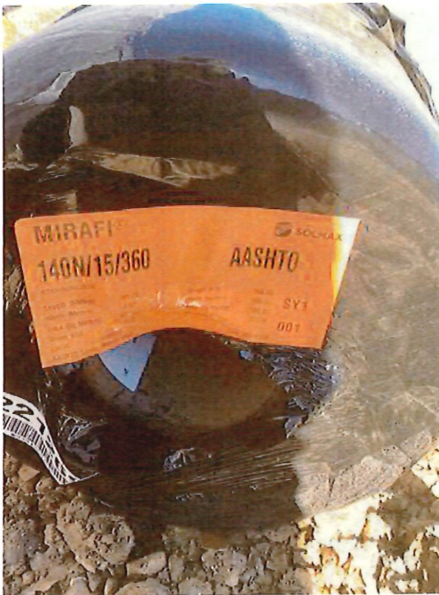
Fabric placed in excavation Ed Carrigan Dec 11, 2024 12:19 PM
