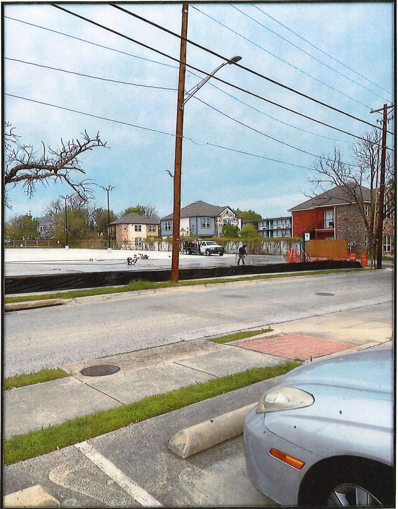
East side of new Parking Lot 59 (former Oak Street Hall site) being power-washed. Silt fencing will remain in place until vegetation can be re-established. View is to the northwest. Wash water was not draining into storm drain curb inlets (03.29.2024).
