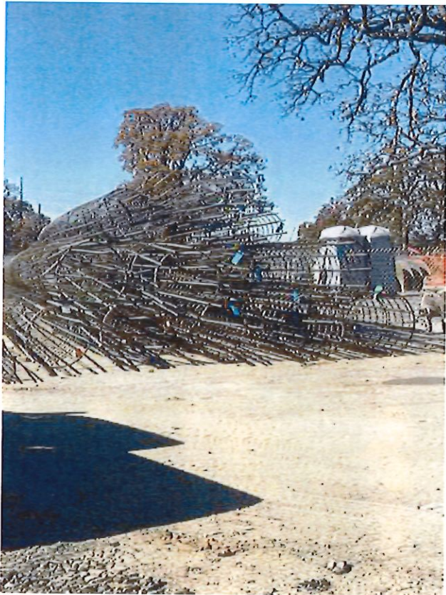
Tied reinforcement cage Ed Carrigan Dec 11, 2024 12:09 PM
