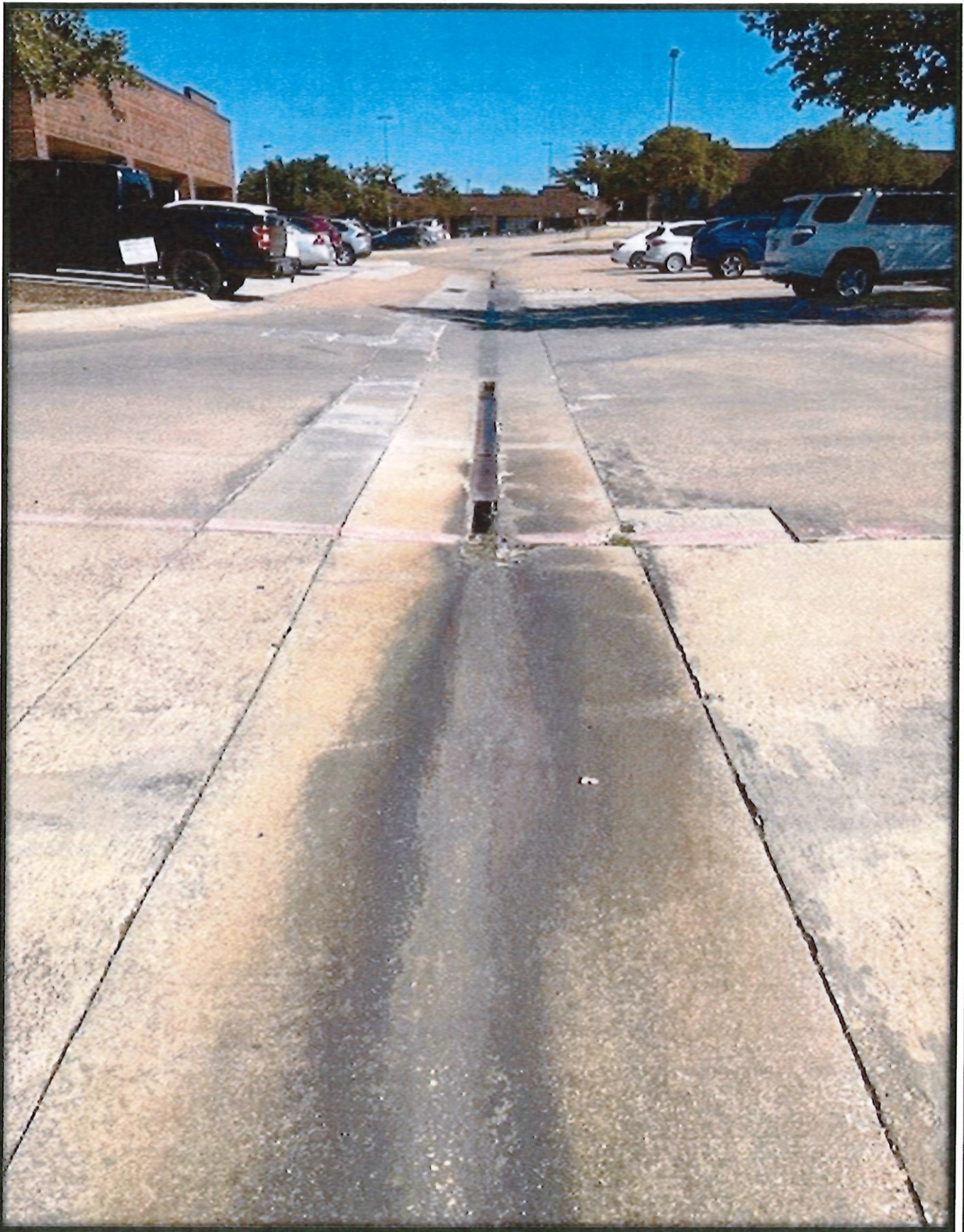
OUT_WHSQ_001: Stormwater flow channel in parking lot of Woodhill Square flowing toward OUT_WHSQ_001. View is to the east.
