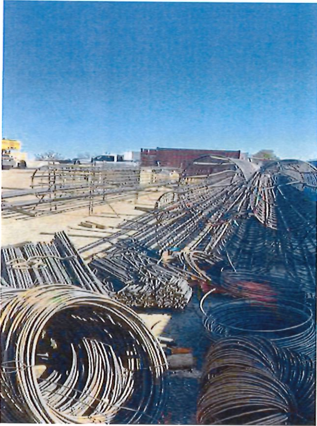
Reinforcement for piers staging/assembly area Ed Carrigan Dec 11, 2024 12:12 PM
