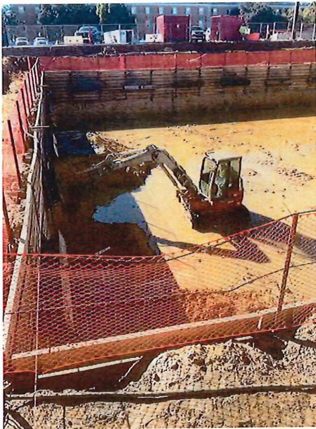
Berkel trimming soil for lagging Ed Carrigan Nov 21, 2024 10:25 AM
