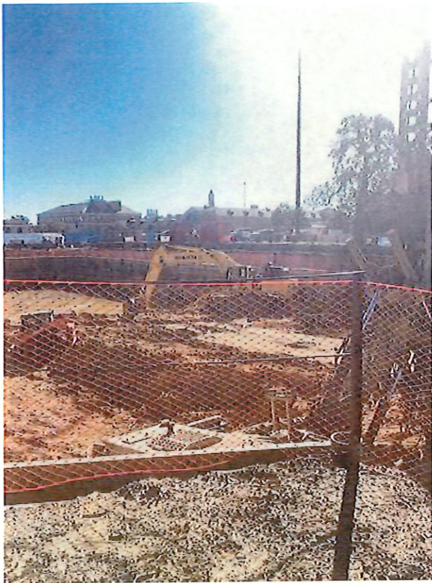
Excavator removing final 5' of soil
