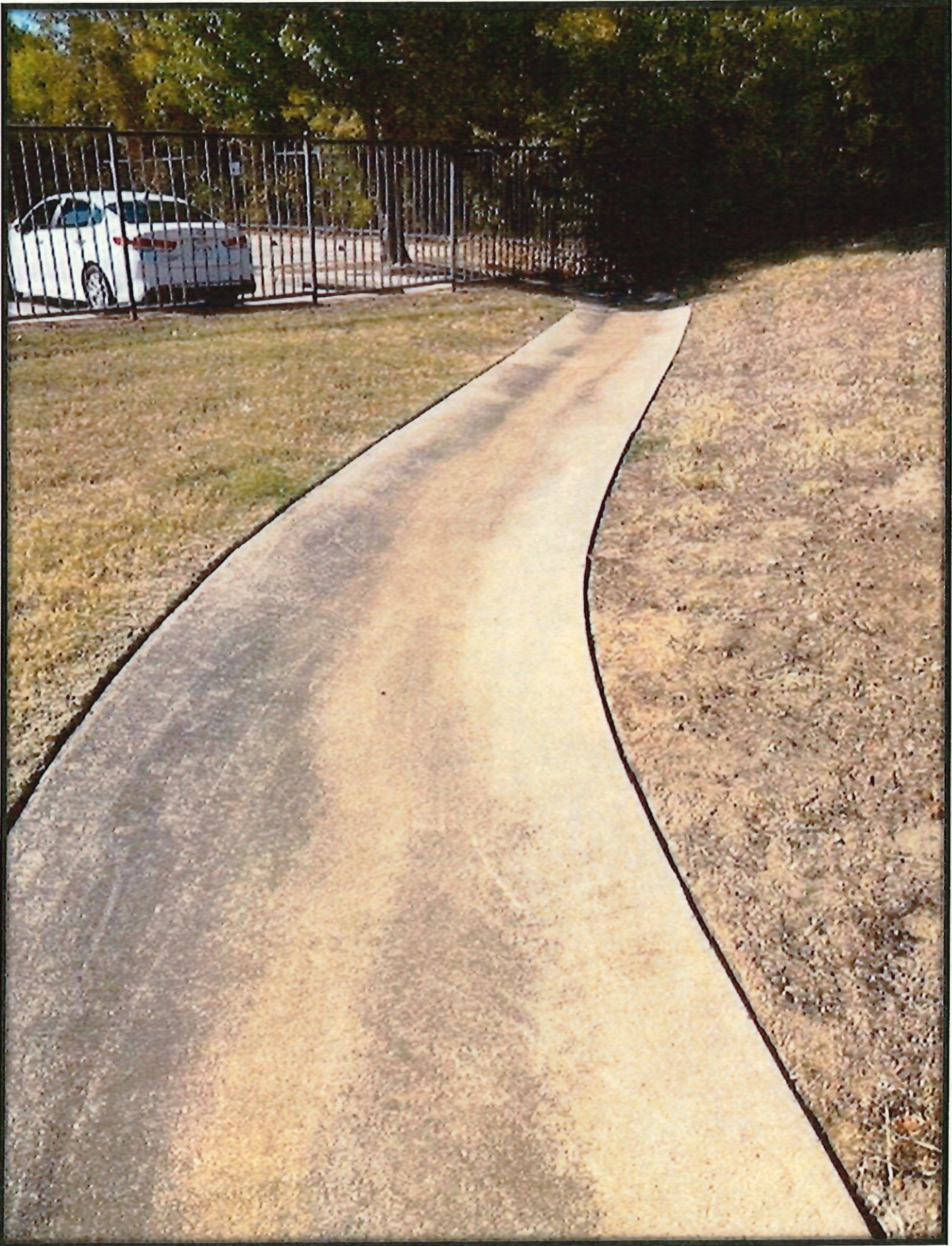
OUT_KFAC_002: Concrete drainage flume along the northwest side of the property. The drainage flows under the fence in the background and into a stormwater drainage culvert.
