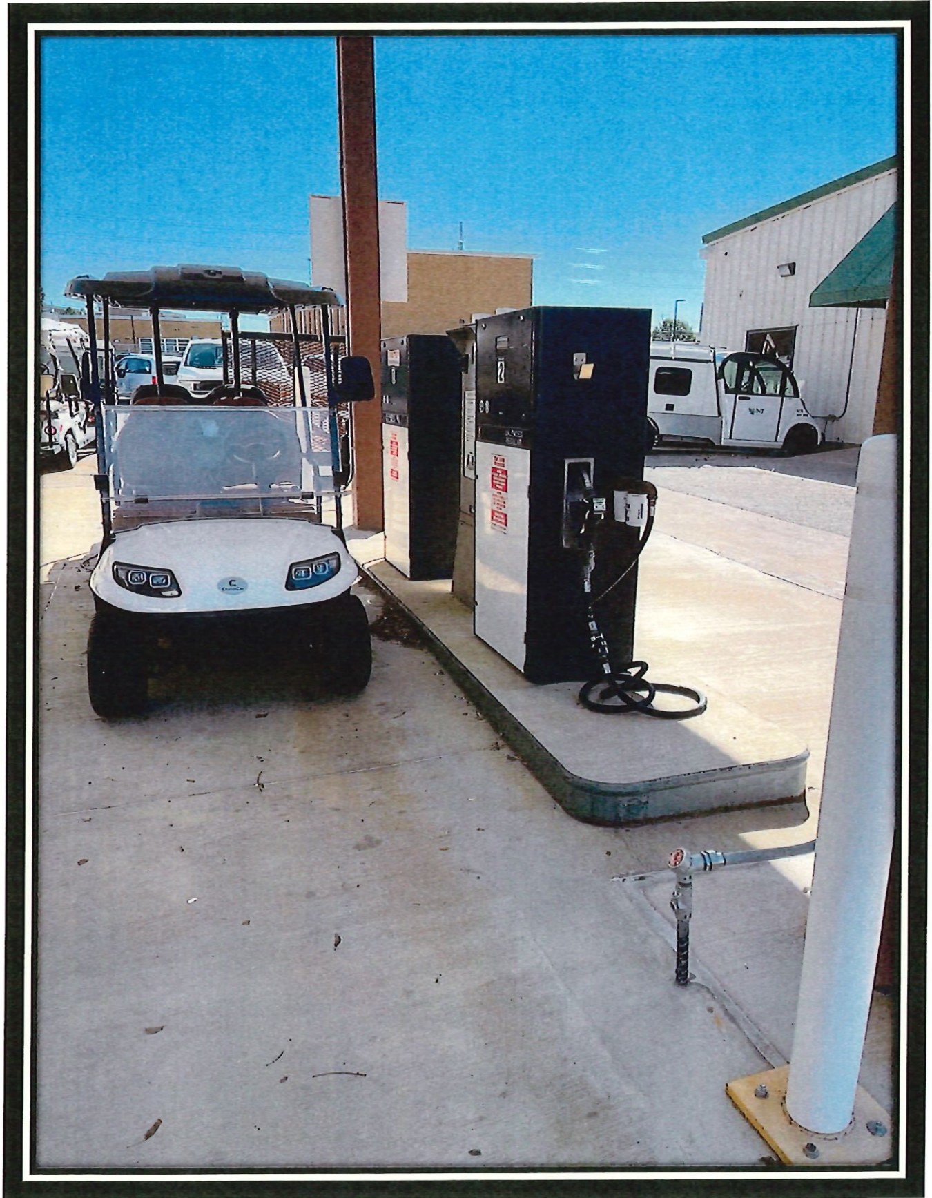
Fuel dispenser pump island outside of Facilities Automotive. The underground storage tank (UST) and the dispenser pumps are currently out of service. The UST will be drained, evacuated, and filled with flowable fill in late Fall and over the Winter. The dispenser pumps will be removed and properly disposed.
