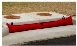
Contain: Contain your work area by isolating debris and pollutants. Containment could include blocking water and/or debris from leaving the area and entering the storm drain. Use gravel bags, sandbags, straw wattle or a silt fence to prevent a potential discharge from leaving the area.
